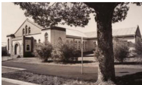
The new church building and hall constructed around the existing facilities on the corner of Hume and Herries Streets.
